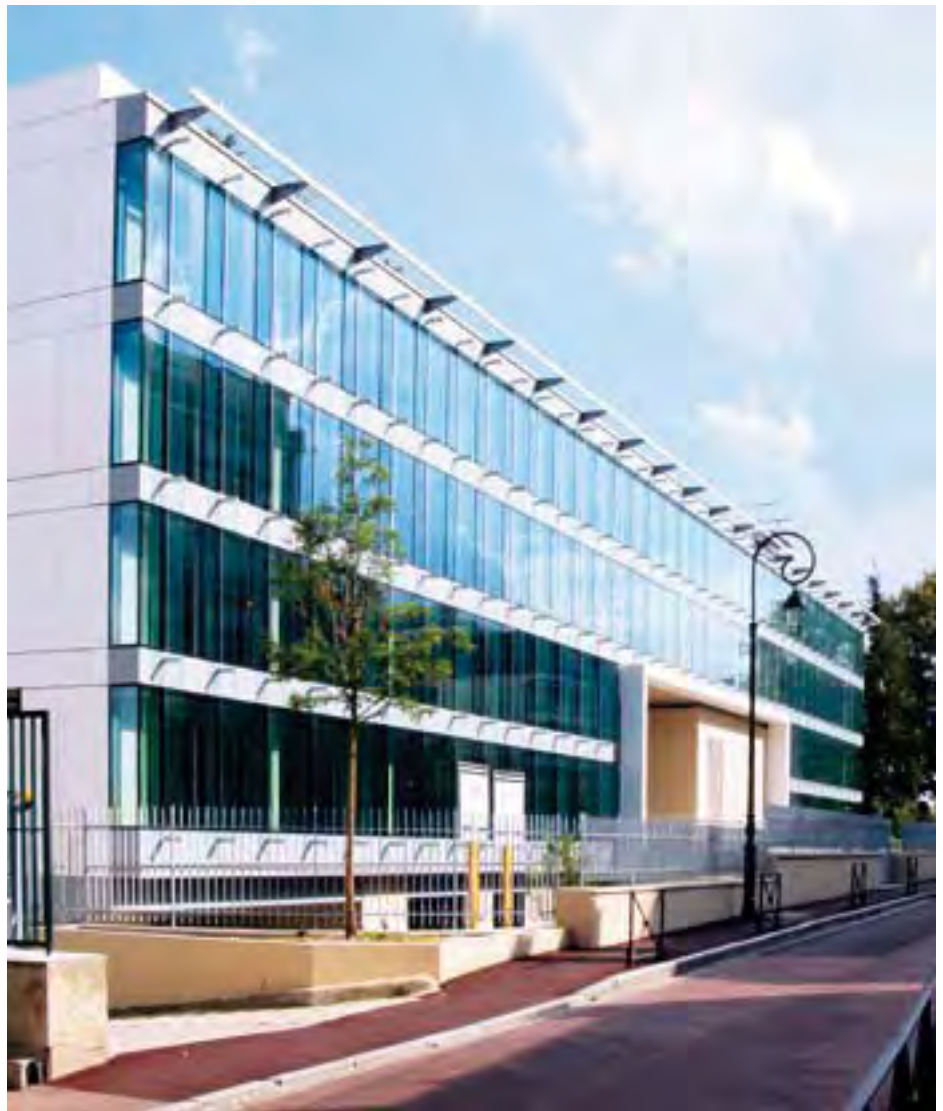
REFURBISHMENT OF THE CLUBHOUSE, Interpol's former headquarters in Saint-Cloud (Greater Paris).
