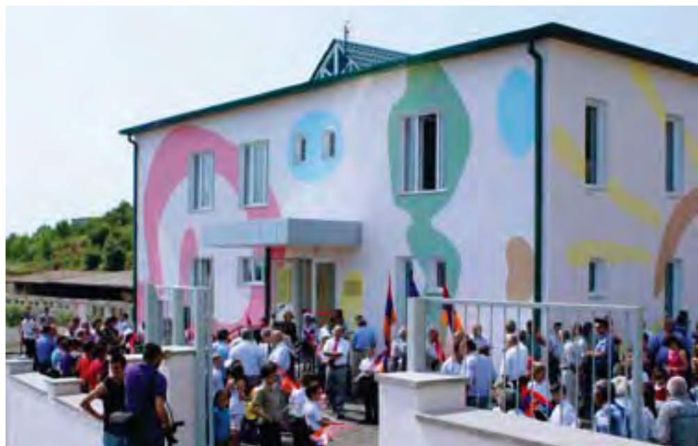
PARTICIPATION IN BUILDING A NURSERY SCHOOL in Armenia.
