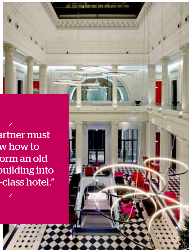
The former Nantes courthouse has been given a second life as the Radisson Blu Hotel, delivered to Axa Real Estate by Altarea Cogedim.
