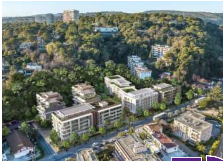
Basement project (Cagnes-sur-Mer)
