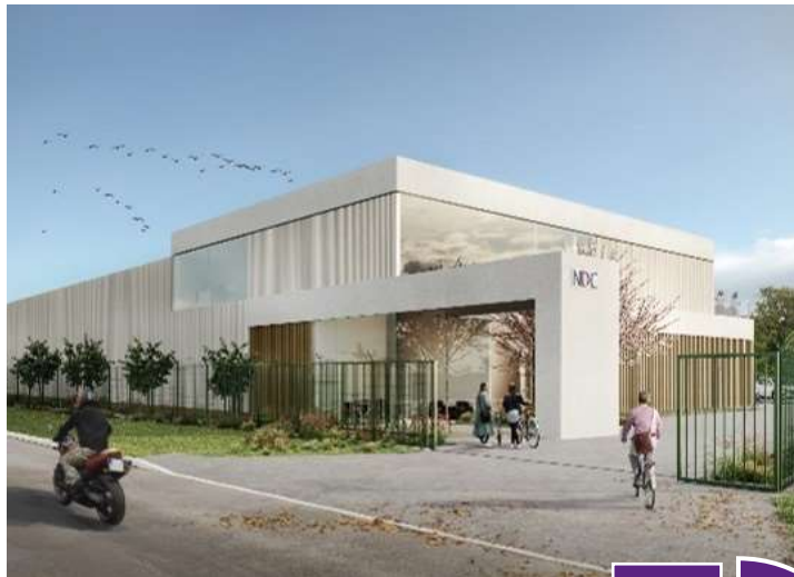
Data center NDC Roazon (Rennes)
