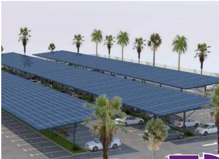
Car park solar canopies
