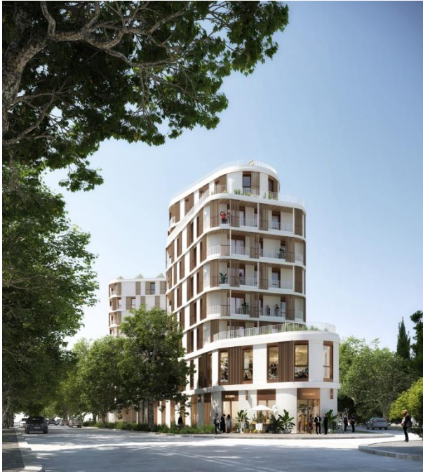
“Flora” building, Nanterre. FPI Pyramide d’Argent award for Low-Carbon Building SIATI award for greenest building of the year.
