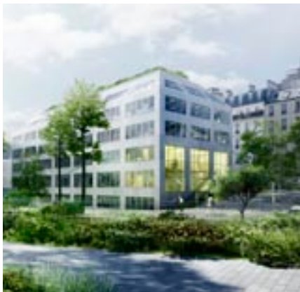
At the heart of the Pajol urban renewal zone, Green One is the first building with a BBC level of energy performance in Paris.
