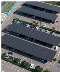
Ombrières parking de centres commerciaux
